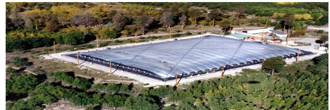
Fig. 1. Aerial view of the Milagro pond with the light-tight cover inflated for work inside..
